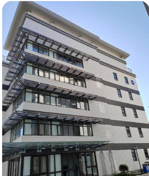
Kunshan Campus Integrated Building
