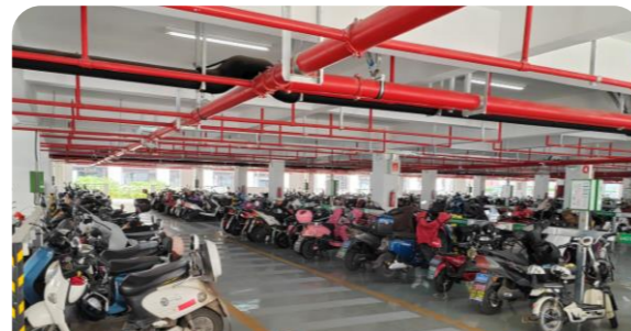
New parking building with 1,097 electric scooter parking spaces.
